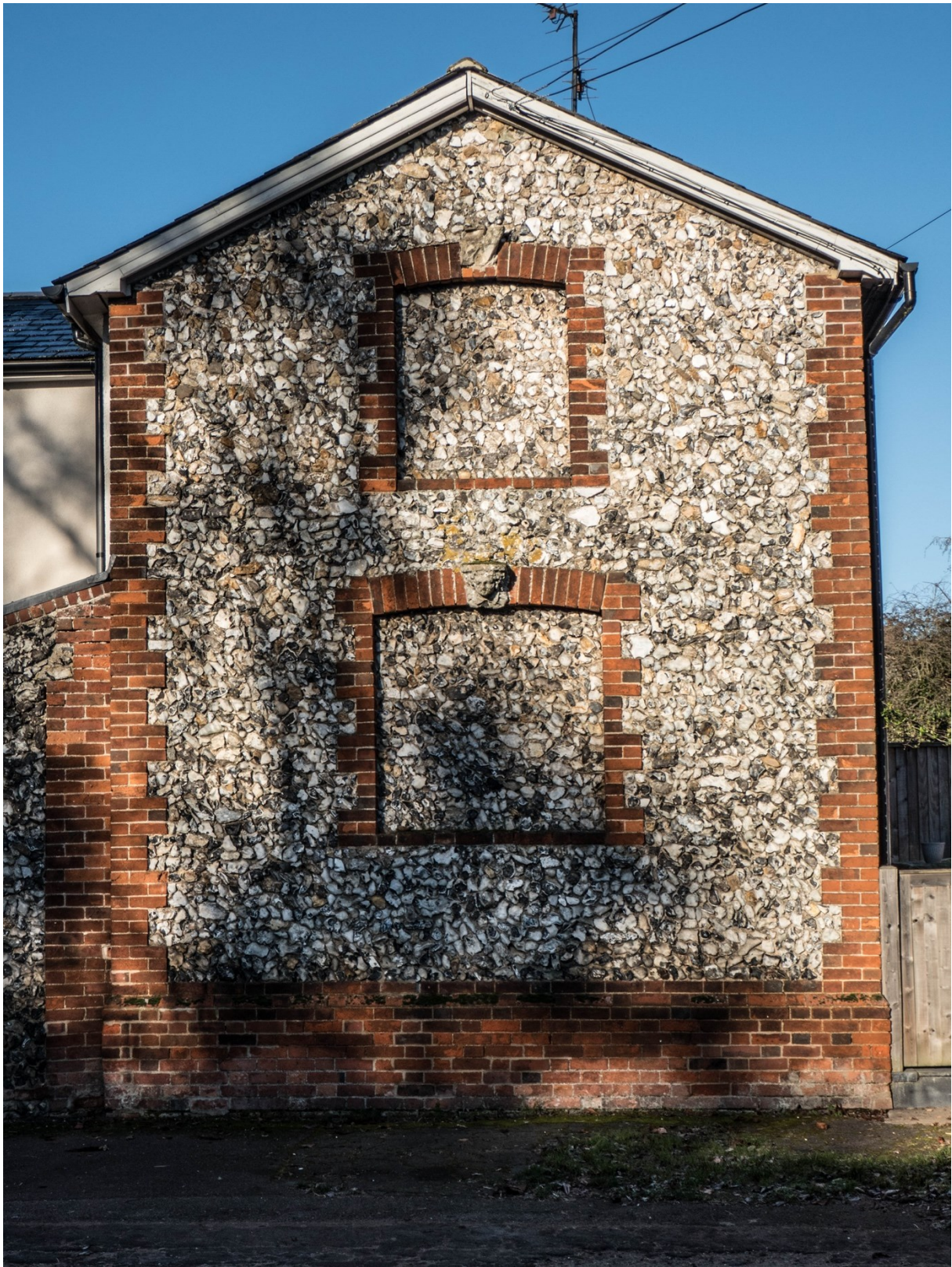
Figure 39: Chestnut Cottages (detail of end wall)
